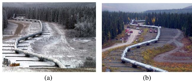
**Fig. 1:** Trans-Alaska Pipeline on slider supports where it crosses the Denali Fault [6]. This pipe suffered some damage, but no oil spills occurred. A large arc in the pipe can be seen in image (b), due to shortening of the zigzag-shaped pipeline trace in the fault zone.
